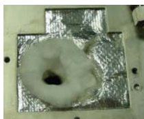
Figure 3.12. Cut into the Insulation
